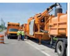
through several filter systems parked onsite and then sent back into the drain to be used to remove the sediment from the next segment of the siphon pipe.
