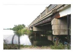
The Road Commission for Oakland County (RCOC) looking to replace the was superstructure on this bridge. The Federal Sufficiency Rating had dropped below 10, and the bridge was in need of repair. SDA was selected in 2006 to complete the design. When the structure study was completed, it was determined that the bridge substructure would not be able to handle the increased dead loads due to the increased deck width and changes in design criteria. The most economical
