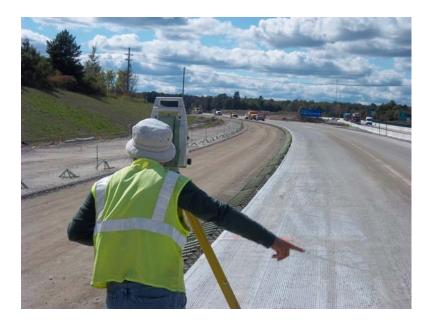
**Preparation prior to staking** included review of the plans, computing **stakeout points**, preparing **cut-sheets**, creating detailed **grade books**, and creating a detailed and precise **digital terrain model** for the contractor's use with their GPS machine control system. Stakeout computations were performed in the office using AutoCAD Civil 3D and MicroStation platforms.
