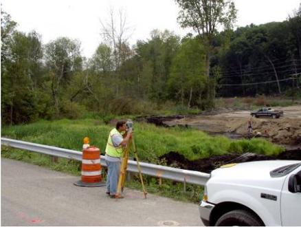
**Spalding DeDecker Associates, Inc. (SDA)** provided construction staking. This project was METRIC. Special Provision based on the Michigan Department of Transportation's, "1990 Standard Specifications for Construction," which was modified to apply to a metric project, was used. A special provision provided the guidelines for WCRC staking requests.
