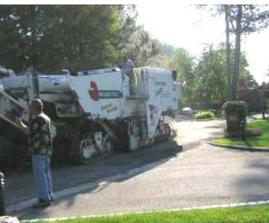
Construction consisted of adding/upgrading storm sewers and drainage structures, crushing and shaping existing asphalt pavement, placement of a 6" aggregate base, placement of 2' concrete curb and gutter, and paving with 4" of asphalt. There were also minor improvements to the Commerce Road and Seminary intersections and drive approaches.
