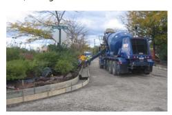
**Spalding DeDecker Associates, Inc. (SDA)** provided design and construction engineering services for the reconstruction of Crowe and Ingersol Drives in the Town Center area of the City of Novi. This project included the removal of an aging concrete roadway with integral curb with new concrete curbing, asphalt pavement, drainage structure repairs, new edge drain, and ADA sidewalk ramp reconstruction through a busy commercial area. This City of Novi Capital Improvement
