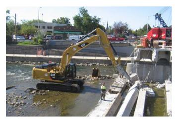
The Macomb Bridge project, over the River Raisin, involves the complete replacement of the bridge superstructure, including deck, beams, sidewalk, railings and approaches, as well as, rehabilitation of existina substructure. After a careful study of the stability of the piers, it was determined that they, for the most part, will
