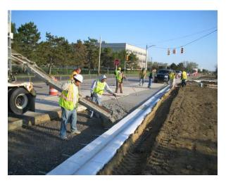
SDA provided construction engineering services and full oversight for the rehabilitation Stephenson Highway. Construction consisted of 1.89 miles of pavement removal, earth excavation, concrete base course, concrete curb and gutter, storm sewer, hot mix asphalt resurfacing, signal upgrades, and drainage improvements. Lane closures were utilized and traffic flow was maintained for duration of the Project.
