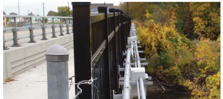
Piping located along the bridge carries the liquid de-icing agent to the high-pressure spray nozzles (below)
