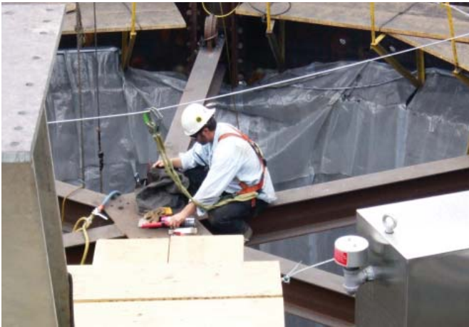
Nearly 200' above the ground, Crew Chief Mark Andrews carefully checks the blast furnace centerline alignment
