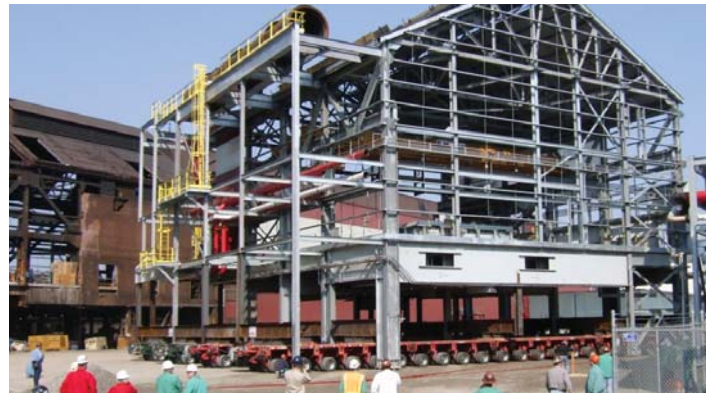
Dozens of onlookers watch as the pre-assembled 1,500-ton casthouse is moved on four haulers to its permanent location.
